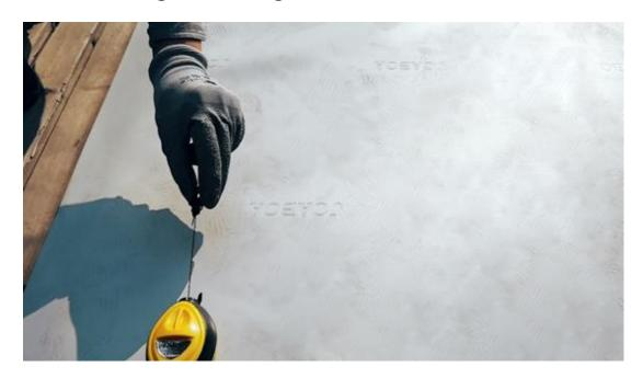
■ Positioning and securing lines to determine the spacing of CS supports in accordance with the design drawings (For design drawings, please contact Sunman).
